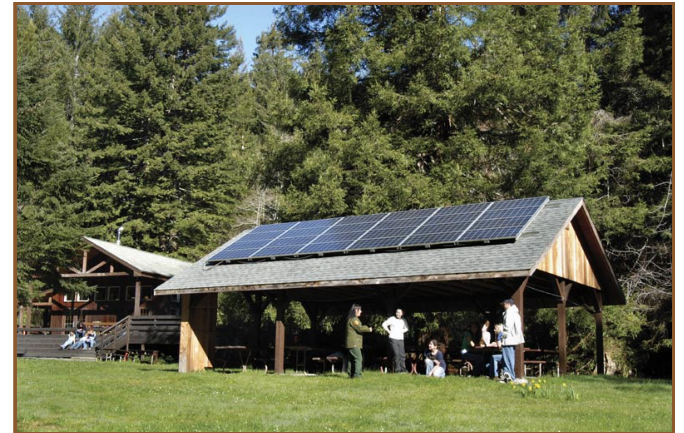
The photovoltaic system at the park's Wolf Creek Outdoor School meets 10% of the facility's annual electricity needs. This is enough energy to provide for half the annual electricity needs of an average home in California.
